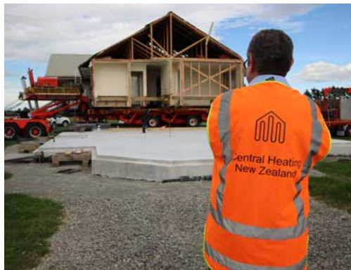
— Relocated home ready for central heating.
