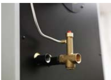
Typical mounting of BVTS when used as water boiling protection
