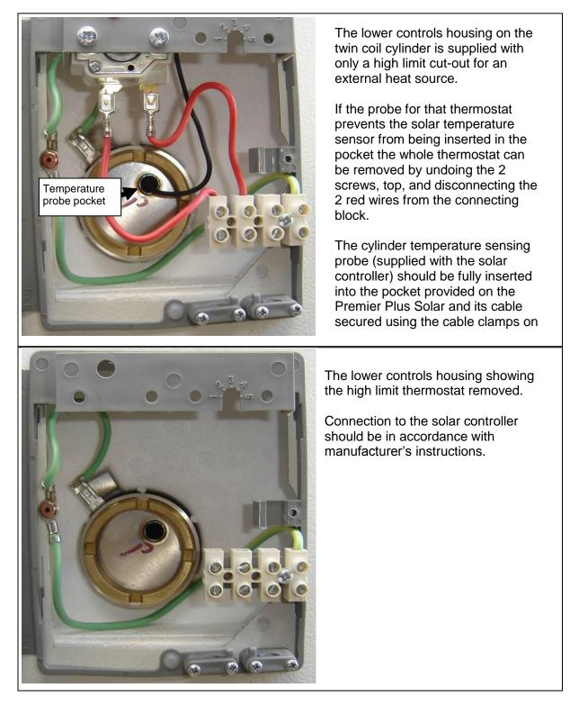
Both coils can be connected together to make one long coil for faster reheat. In this case the external heatsource thermostat that comes in the upper controls housing will need to be moved to the lower controls housing.
