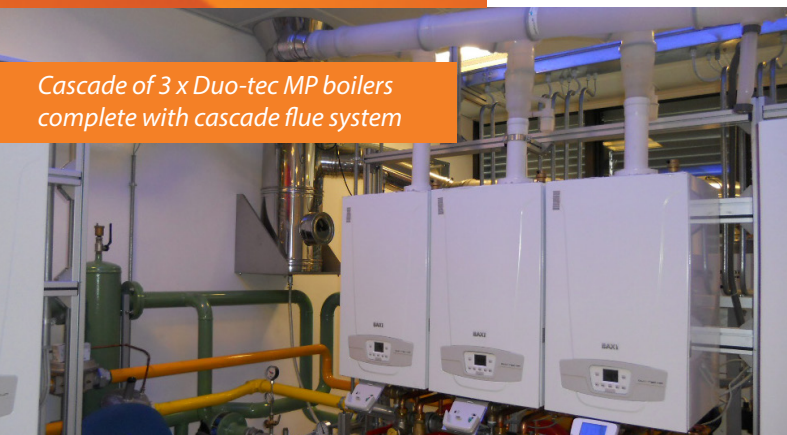
900kW Baxi Power HT gas boiler cascade
