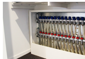
— Underfloor manifold cabinet tucked away in a closet, with cover removed
