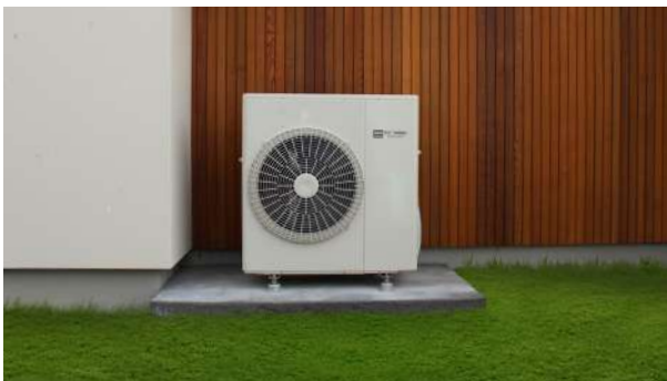
Option 3: Change the boiler out for a Heat Pump
