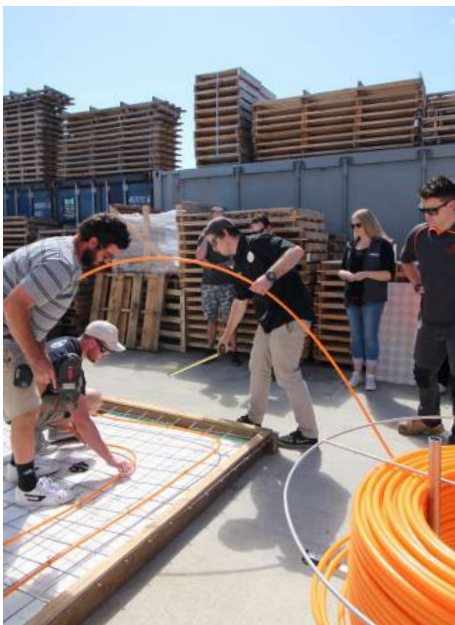
— Inslab underfloor installation training
